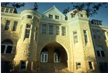
Bethel College Administration Building
