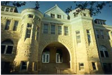
Bethel College Administration Building
